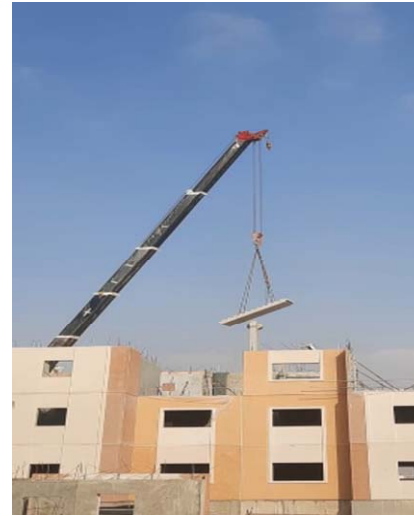
Erection of Stair
