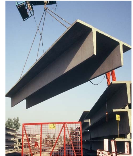
Erection of Double TT
