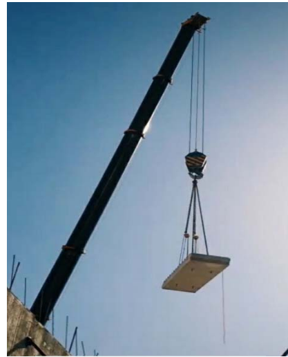
Erection of Hollow Core
