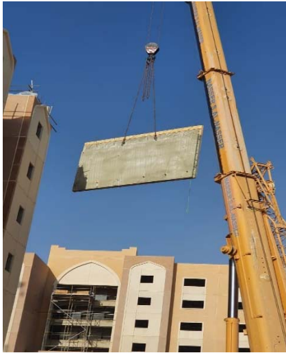
Erection of Panel
